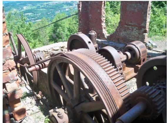
Dual 75-Horse Power engines used to power the railway. A fire scorched the engine house.
