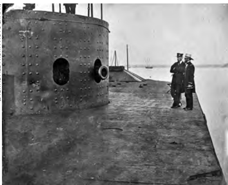
Two men observing the light damage caused to the turret of the ironclad USS Monitor during her fight with the Confederate ironclad CSS Virginia , March 9, 1862, at the Battle of Hampton Roads.
