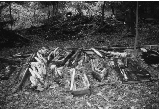
Figure 9: Pink House fragments at Boscobel during salvage efforts in 1997. Image by Charles Lyle, courtesy of Boscobel House and Gardens, Garrison, NY
