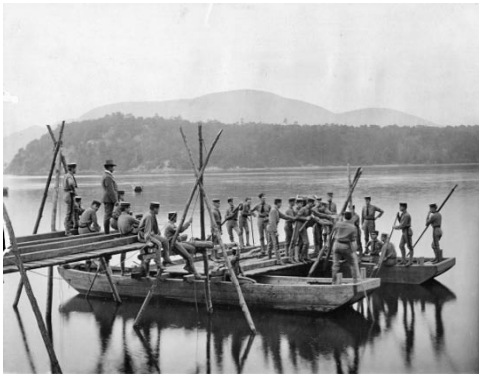
Cadets building a pontoon bridge on the Hudson
