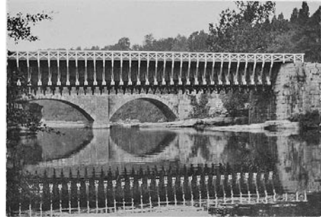
Both of the High Falls aqueducts over Rondout Creek. The 1825 stone one is in the background; the 1847 suspension aqueduct, designed by John Roebling, is in the foreground.
