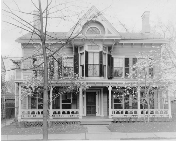
Laura Wylie's house at 112 Market Street, which now houses the offices of the Hudson River Sloop Clearwater.
