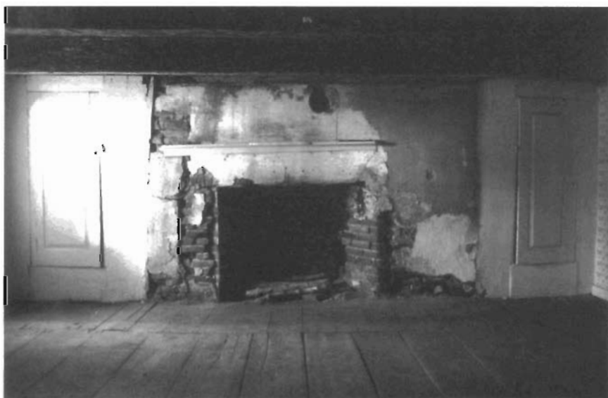
First Floor, west room, west wall, with fireplace.
