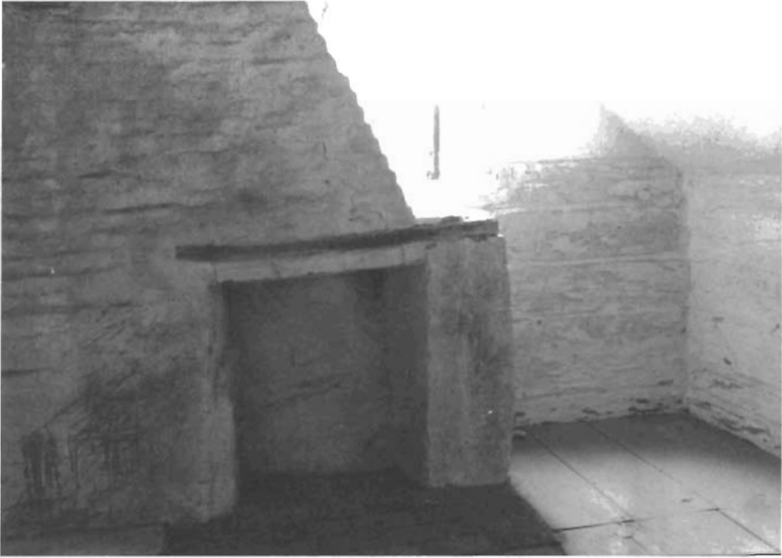
Second Floor, fireplace.
