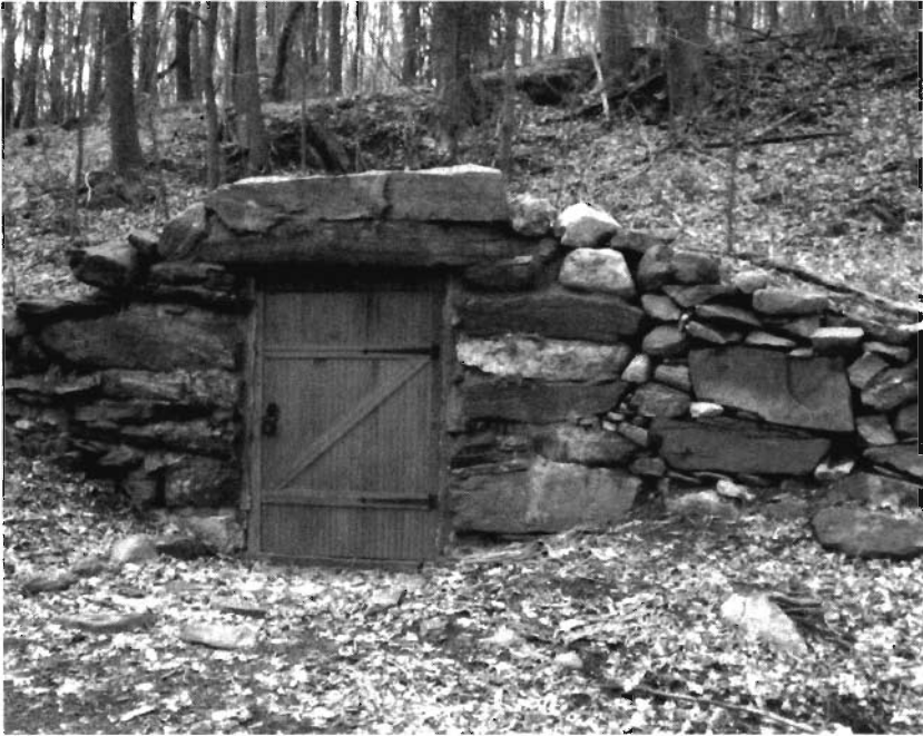
Thick wooden doors were opened or closed, depending on outside weather conditions, to regulate the temperatures in the chambers, believed to have been used as "primitive refrigerators."
