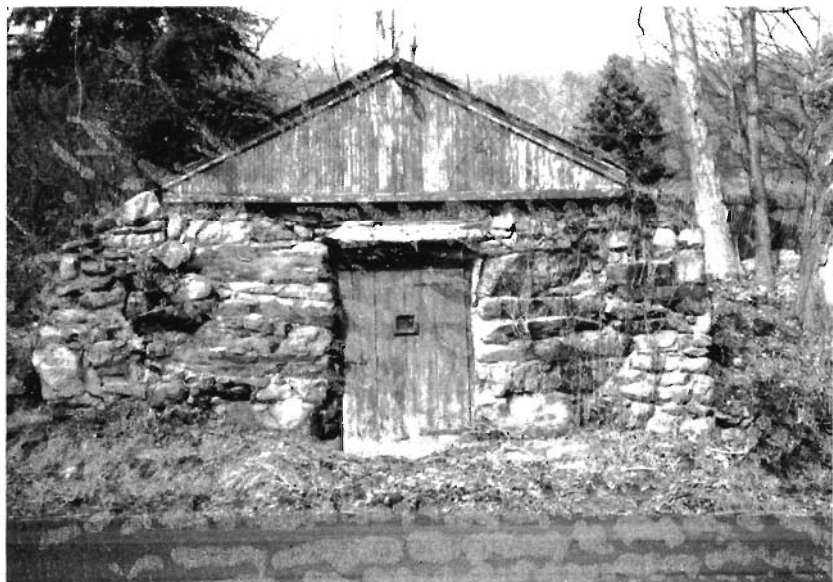
Most chambers did not have wood-framed roofs such as this one. This roof served no purpose and was only for decoration.
