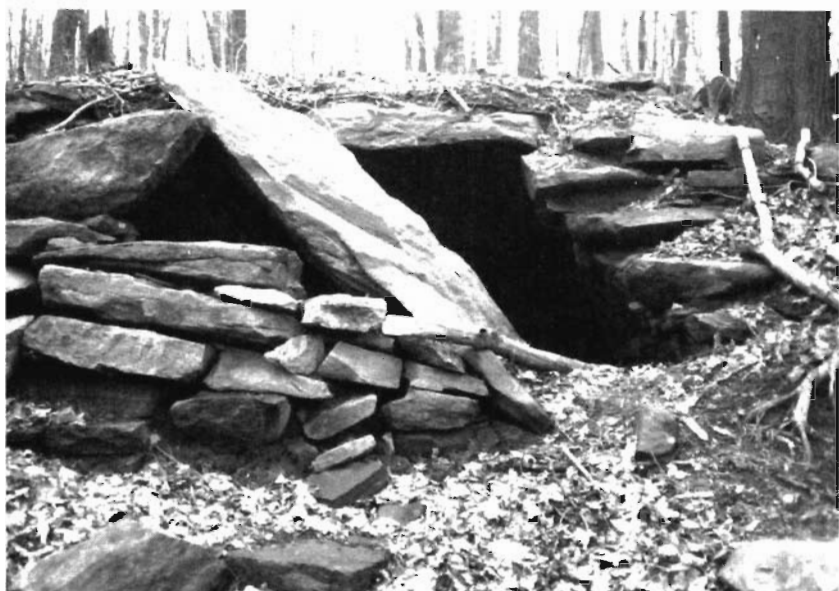
The weight of the stones used to build the chambers leads historians to believe that the early settlers built the chambers since they had the manpower and oxen to move them. Shown here is a roof collapsing from the weight of the large stone slabs.
