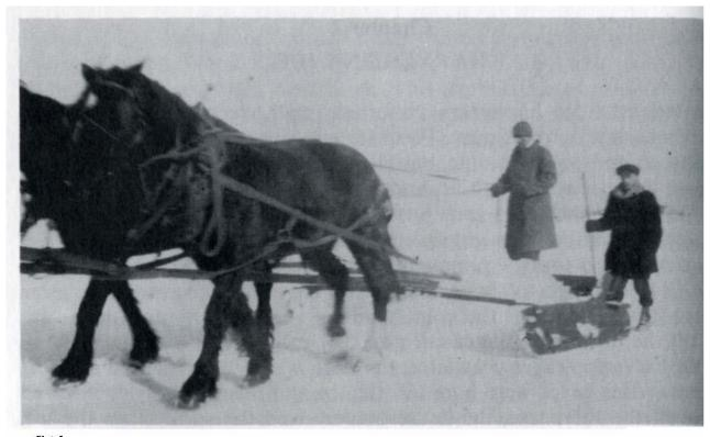
Photo 5 A team clearing the ice field with a snow scraper. Photo Credit: Ice Harvesting in Early America - Hill 10
