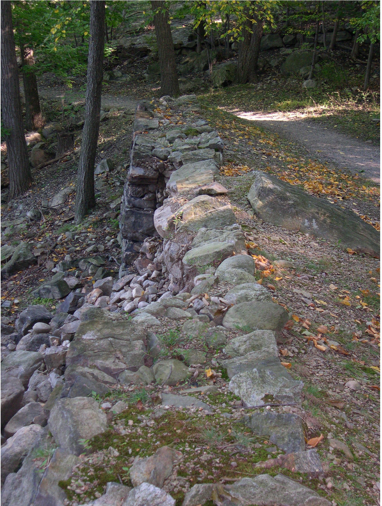
Collapse from Top of Parapet Wall
