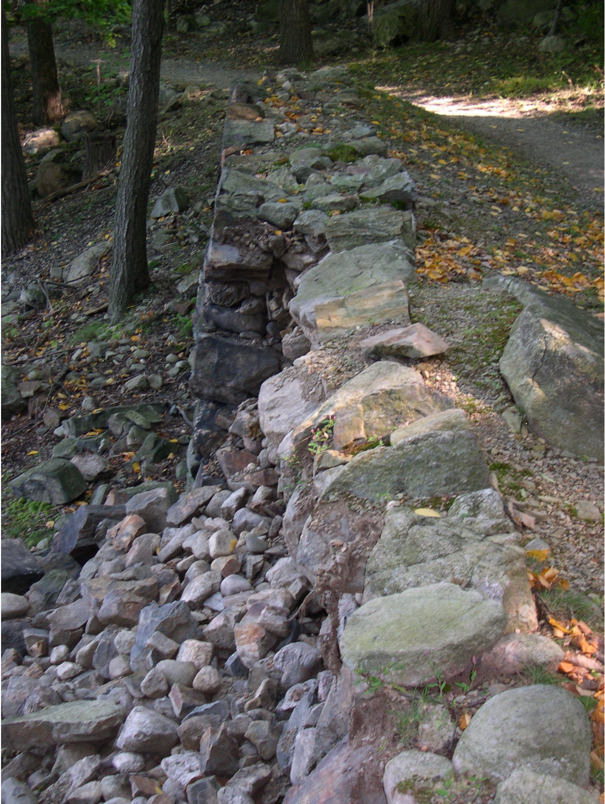
Detail Collapse from Top of Parapet Wall
