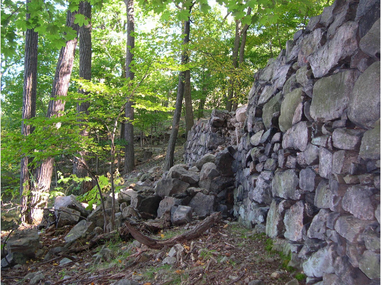
Collapse, Parapet Wall Perspective
