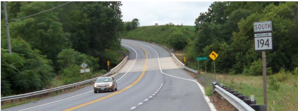
Crossing of the Large Pipe Creek
