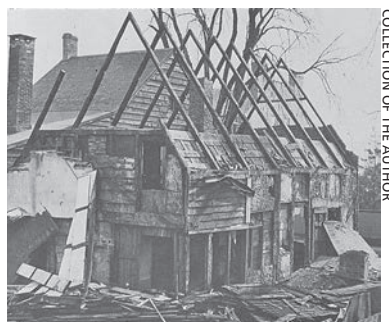
Figure 2 The razing of the Bradt house, Schenectady, in the late nineteenth century. The bent system of framing is clearly seen in this view
