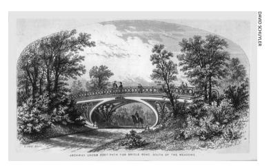
Fig 3: Lithograph of Oval Bridge, a cast iron structure carrying a pedestrian path over the bridle path. This is one of more than twenty bridges that were constructed to provide a complete separation of all forms of traffic. From Board of Commissioner of the Central Park, Sixth Annual Report (New York, 1863)
