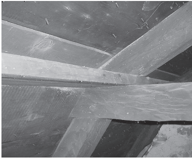
Figure 14 Detail of gambrel framing in the Douw Fonda house, Cohoes (2004)
