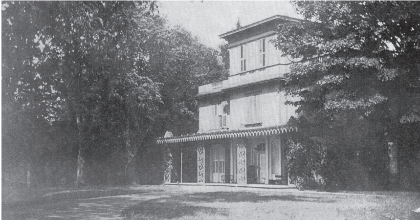
The west façade of the Plumb-Bronson house as redesigned in the Italian Villa style in 1849
