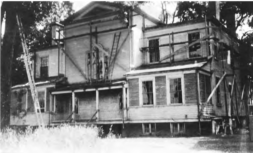
A view of Boscobel house before it was dismantled
