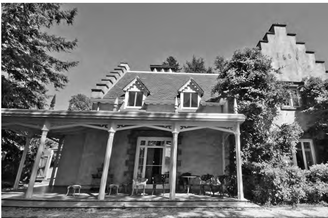
The porch on Sunnyside facing the Hudson River. Photo by Bryan Haeffele, courtesy of Historic Hudson Valley
