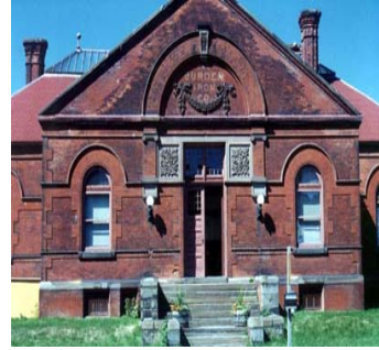
Burden Iron Works Museum
