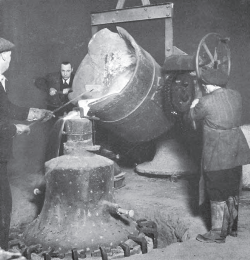
Pouring a cast at the Meneely Foundry, c. 1937
