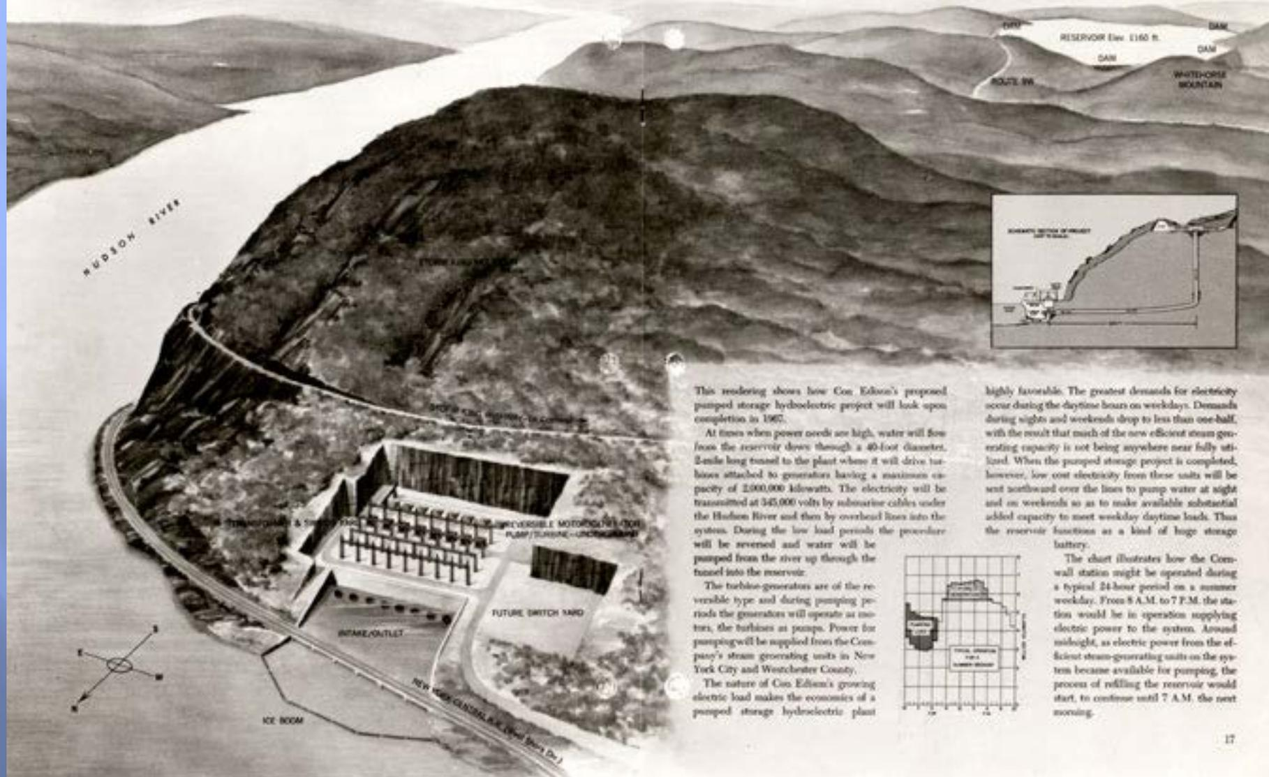
This rendering shows how Con Edison's proposed pumped storage hydroelectric project will look upon completion in 1967.
